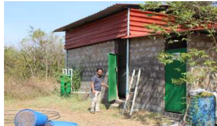
Biogas bag and Compressor Room
