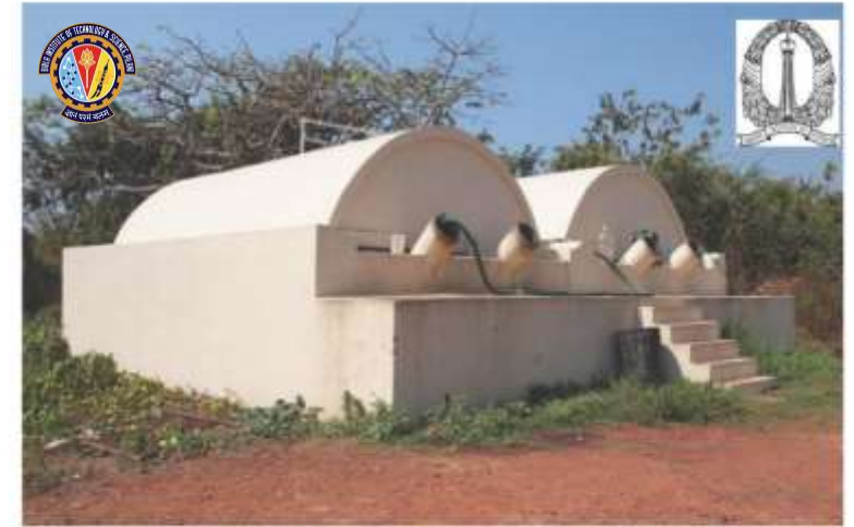
1 tpd plant at BITS Goa Campus, 2009: Mess and kitchen wastes
