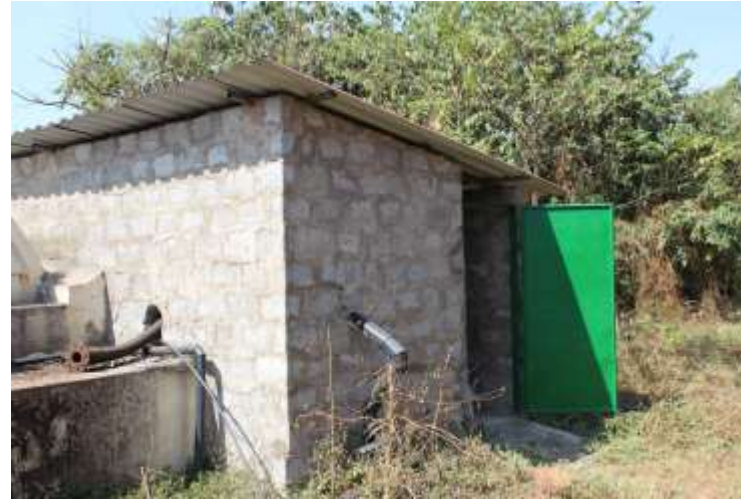
Food waste Macerator room
